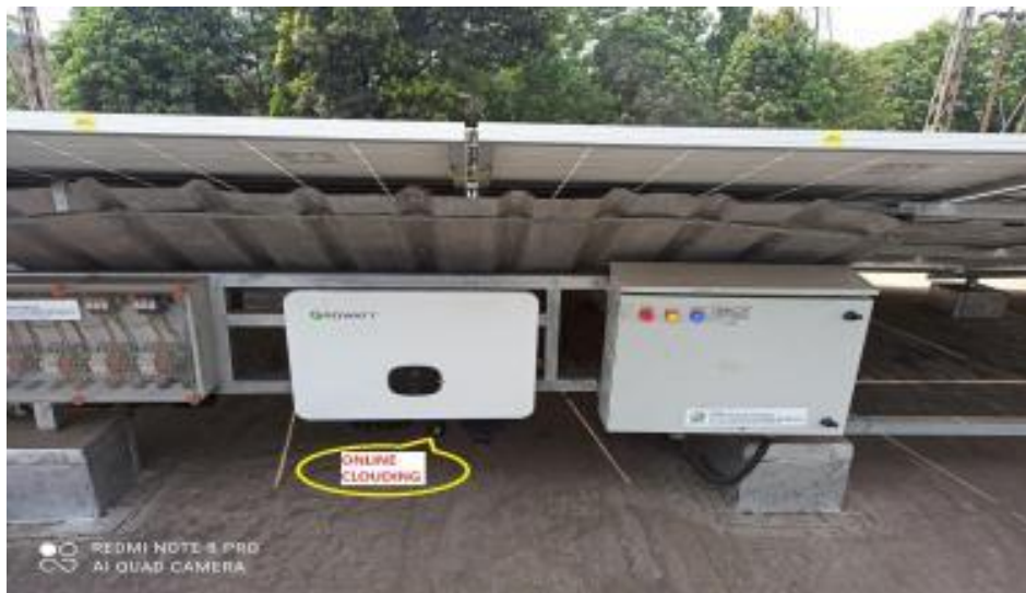
IP65 Inverter with Communication port for online monitoring and daily report
