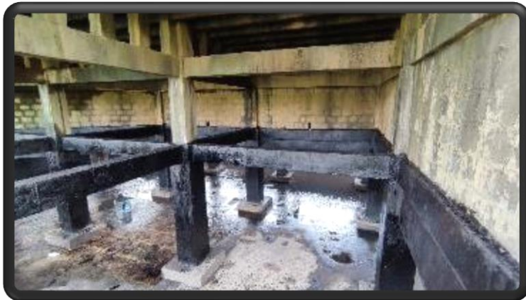
Vacuum improvement by CT cell bitumen coating
