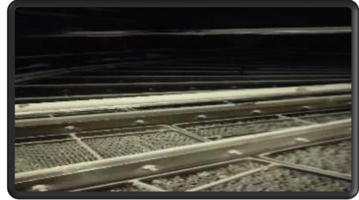
Fan power reduction by APH seal replacement
