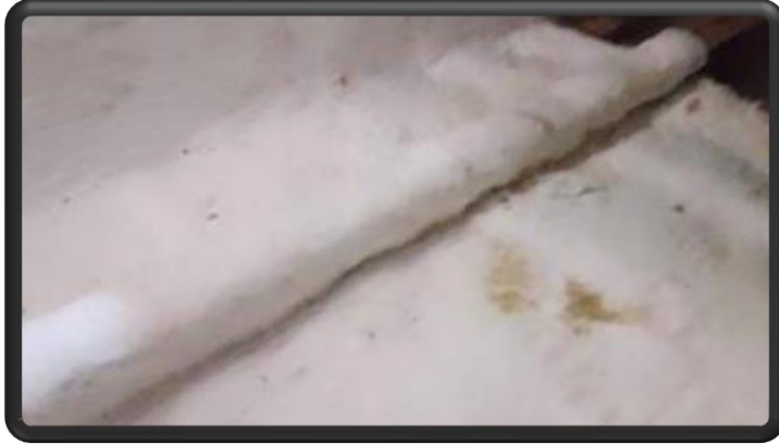
Boiler penthouse cleaning & air sealing
