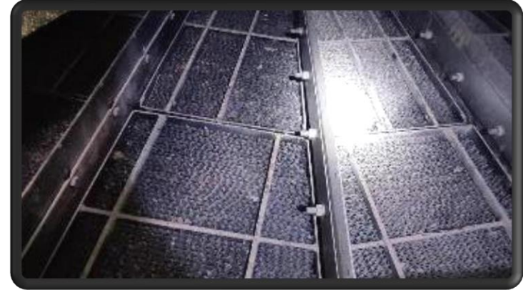
Flue gas temperature reduction by APH basket replacement
