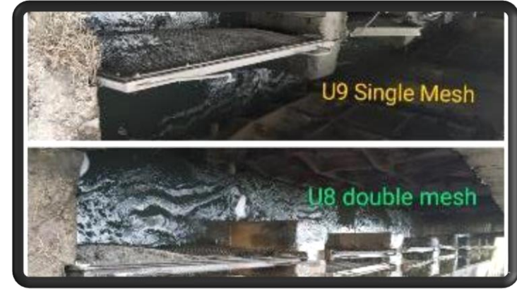
Double layer bucket strainer installation for vacuum improvement
