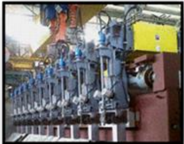
Anode Beam Raising Frame
