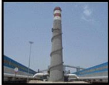
Gas Treatment Centre with Bath recycling and cover mix system
