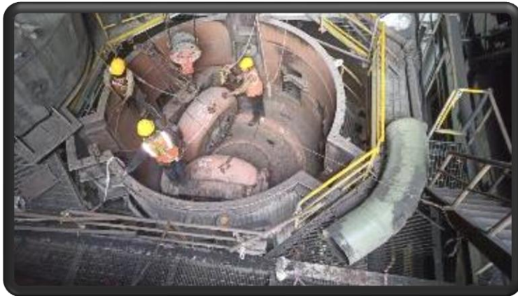
Auxillary power reduction by mill roller replacement
