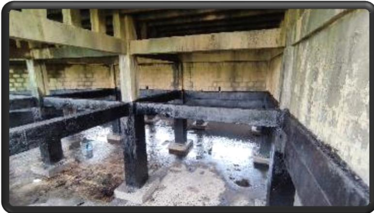
Vacuum improvement by CT cell bitumen coating
