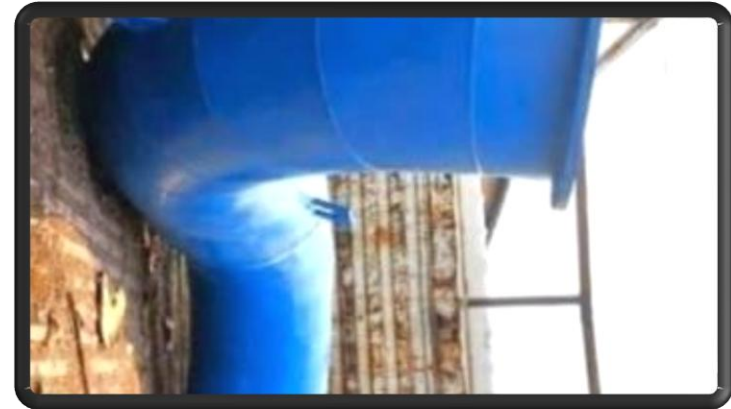
Ceramic coating at coal pipes
