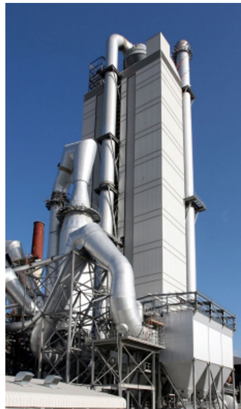
Figure 24: Padeswood Kiln and Cement Plant
