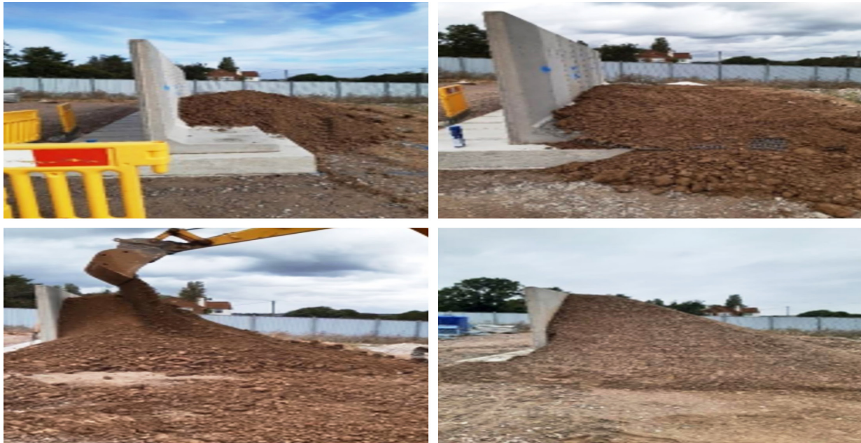
Figure 15: Sequence of backfilling retaining walls with sulphated soil (clockwise from top left)
