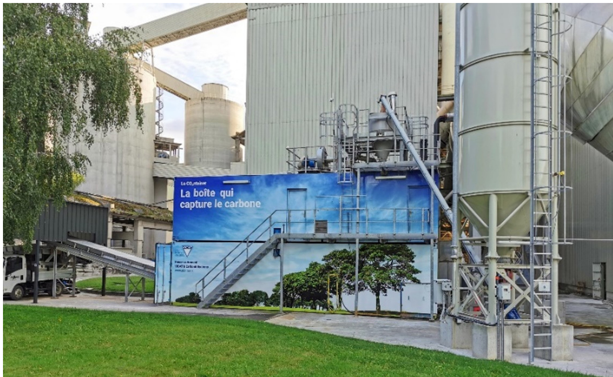
Figure 33: CO 2 ntainer at Vicat
