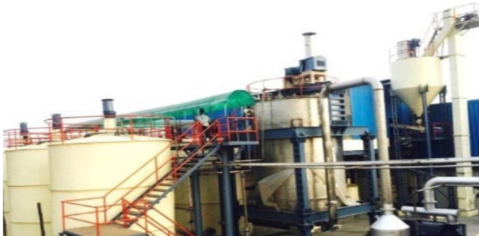
Figure 6 OPM - Onsite PCC Plant
