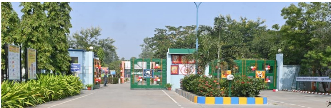
BCML Plant, Haidergarh, Uttar Pradesh
