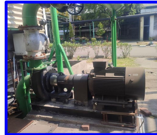
Single Energy Efficient Pump on Cooling Tower Supply Pumps with VFD
