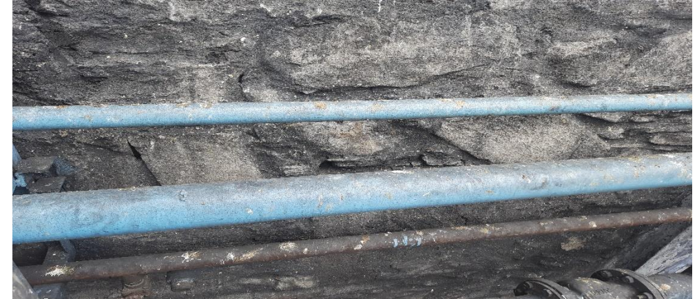
Air Line in Mixing Section Before
