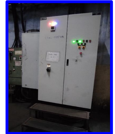
Single Energy Efficient Pump on Cooling Tower Supply Pumps with VFD
