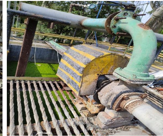
Old Inefficient Pumps on STP section with Fixed Starter Panel
