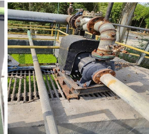
Single Energy Efficient Pump on STP Section Pump with VFD
