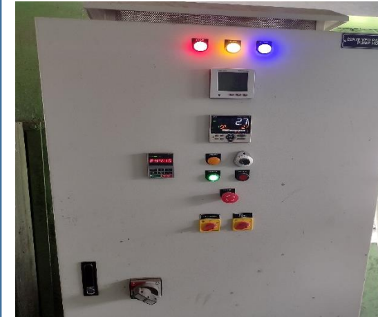
Single Energy Efficient Pump on STP Section Pump with VFD
