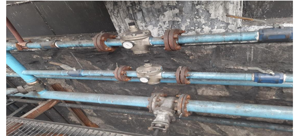
Air Line in Mixing Section After Modification
