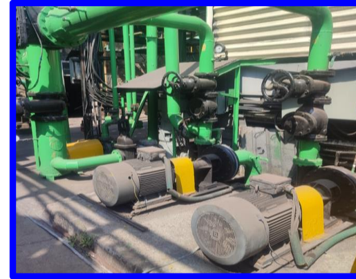
Multiple Pumps on Cooling Tower Supply Pumps with Fixed Starter Panel
