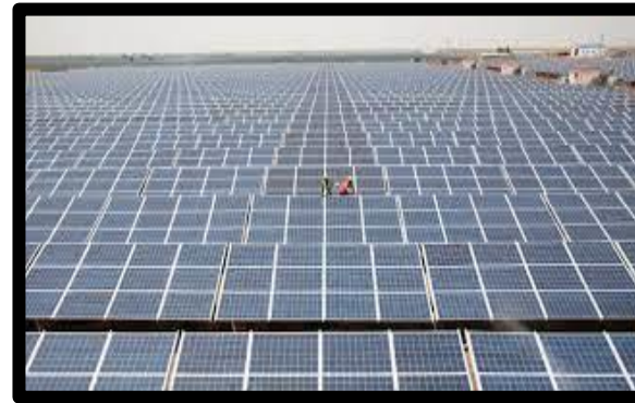
Solar Plant Capacity – 3 MWp
