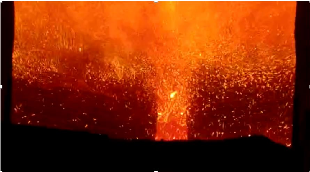
Furnace before use of Oxybooster O2 Swift
