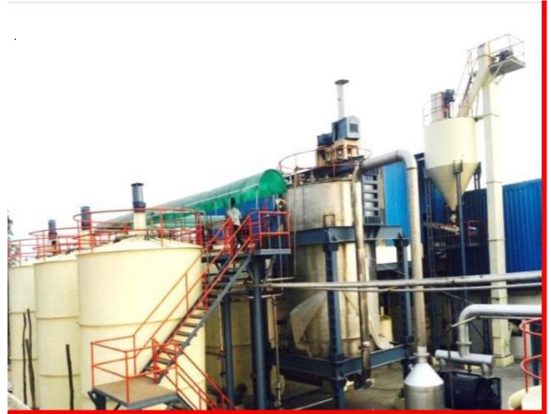
View of OPM - Onsite PCC Plant
