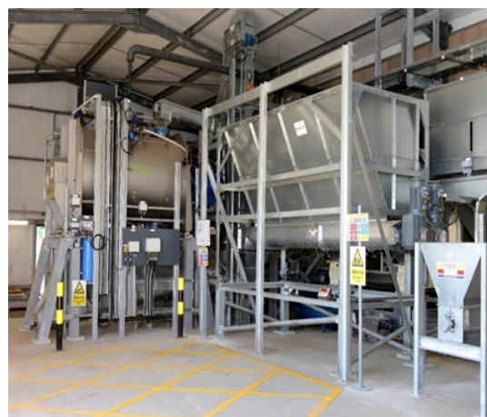
Figure 2: CCm's CO 2 utilisation in the fertiliser production plant at Minworth
