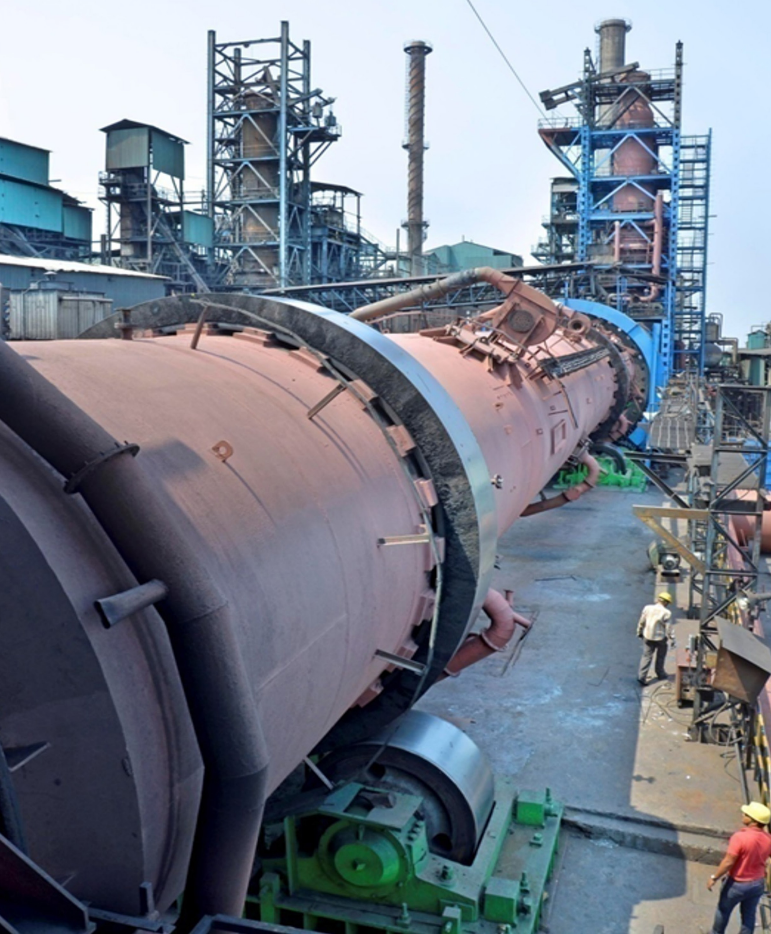
Rotary Kiln at Godawari Power & Ispat Limited's (GPIL) unit in Raipur, Chhattisgarh
