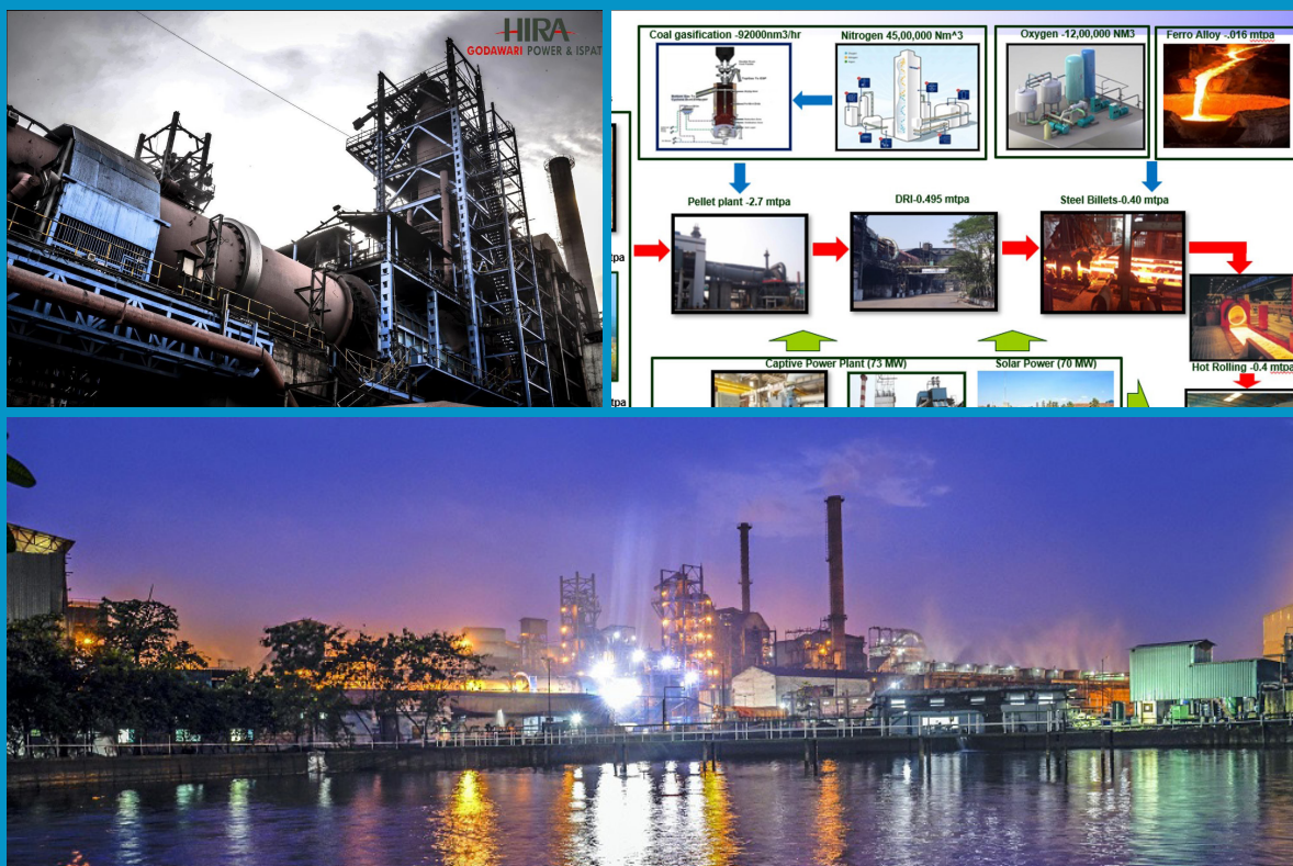
GPIL Plant, Raipur, Chhattisgarh
