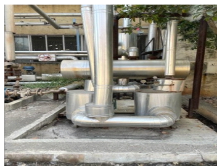
Figure 8: Flash Stream Recovery Pump
