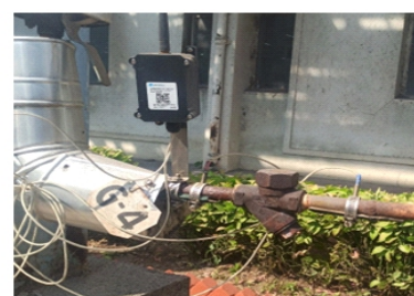
Figure: IoT Based Steam Trap Monitoring System at Raymond Chhindwara Plant
