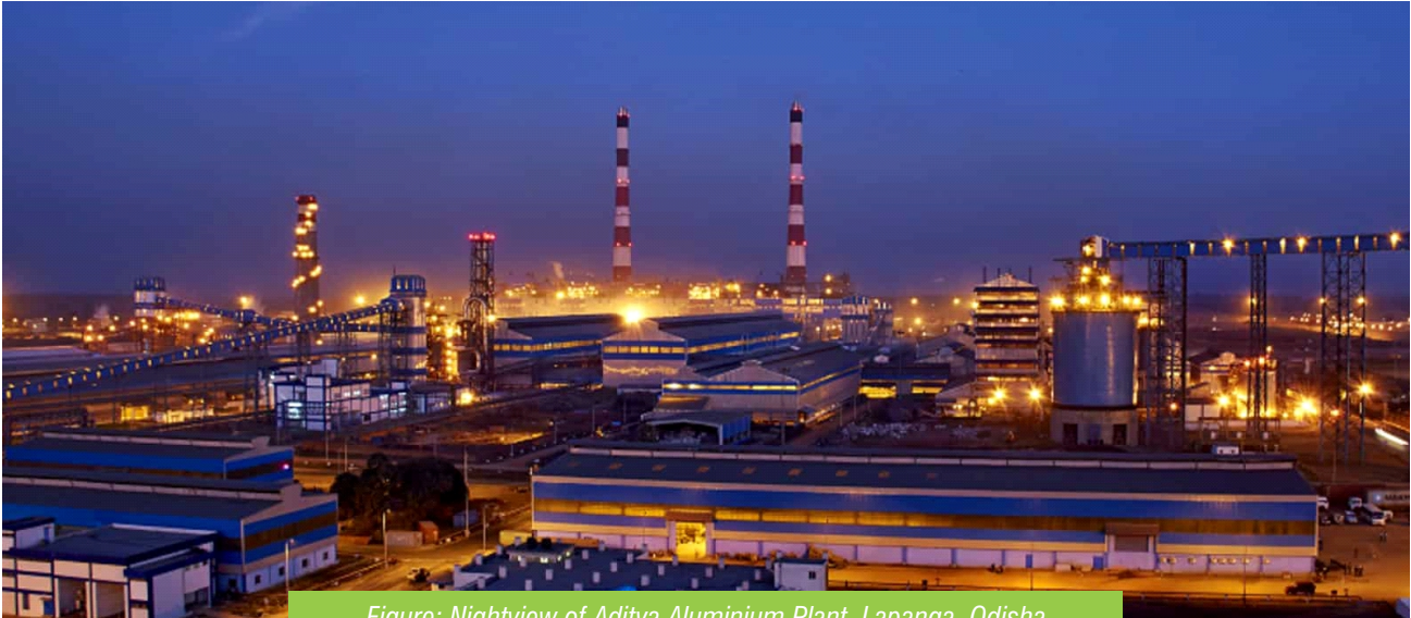
Figure: Nightview of Aditya Aluminium Plant, Lapanga, Odisha
