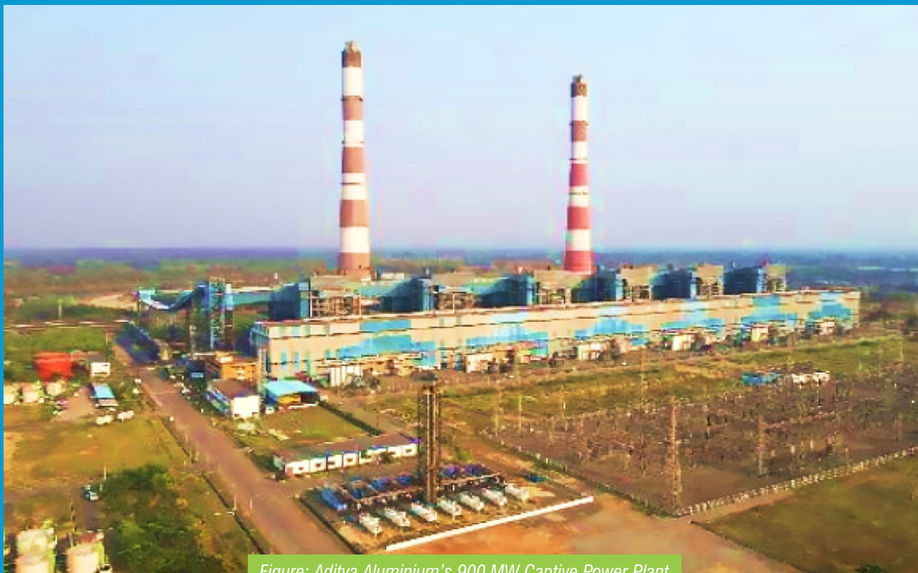
Figure: Aditya Aluminium's 900 MW Captive Power Plant
